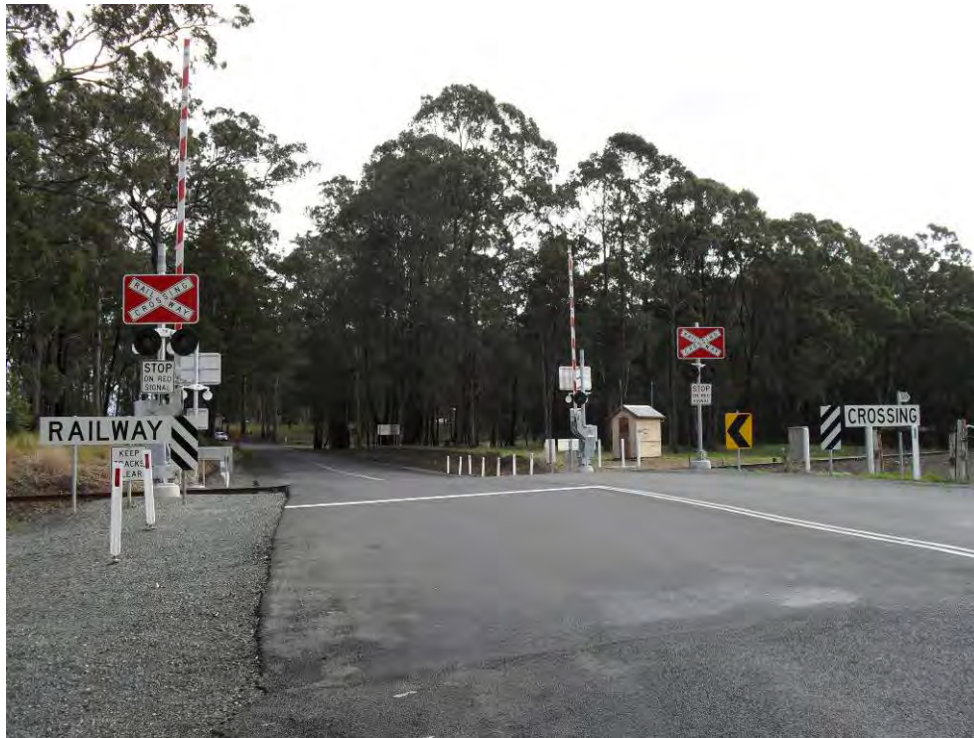
Figure 9.2.9.1: Existing Level Crossing
